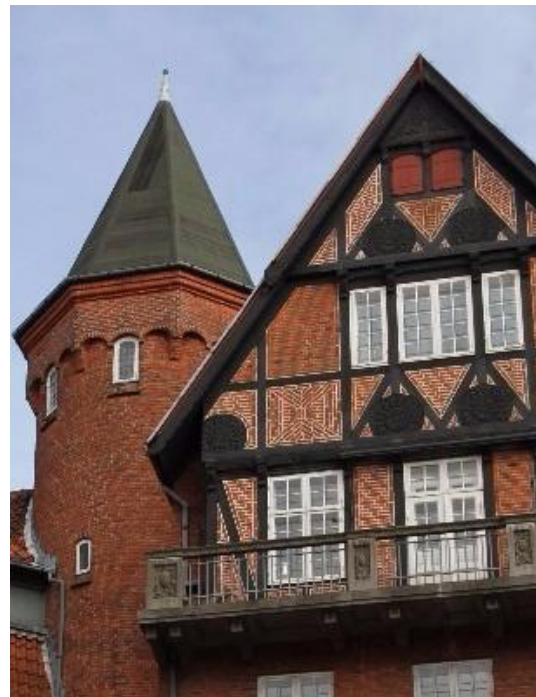
Older buildings are often retrofitted with Internal insulation to maintain the external appearance, but this can create problems such as moisture damage. RIBuild investigates how to install internal insulation in a secure way. Photo: Sirid Bonderup.
