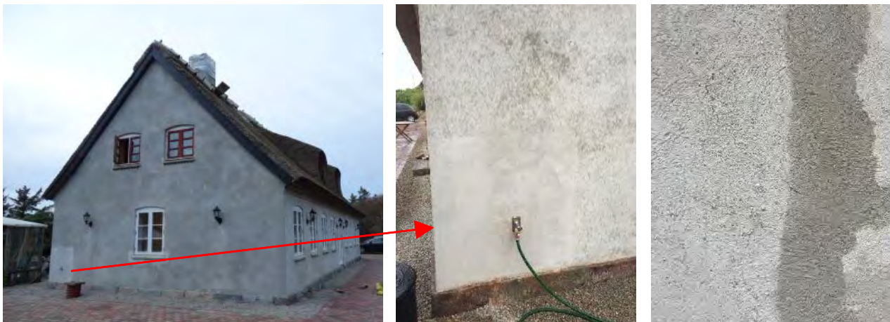
Figure 8-3: Test fields with hydrophobization in 2016. Left: southern gable with 1 m 2 hydrophobized in the left corner; Middle: close up of the hydrophobized test field during rain; Right: water sprayed on the border between hydrophobized and not hydrophobized area of the façade.
