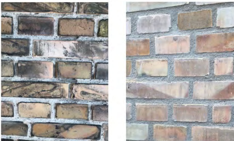
Figure 9-4: Before (left) and after (right) refurbishment and hydrophobization
