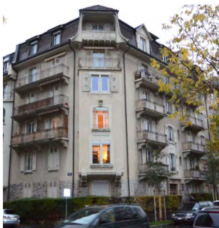
Figure 76 North-east view of the building
