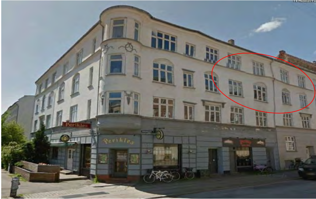
Figure 45 Kildevældsgade 69, Copenhagen, Denmark, with indication of renovated apartment
