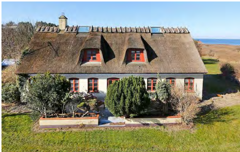
Figure 51 Klitgården, East facade
