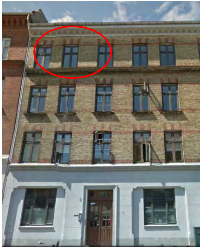
Figure 48 Thomas Laubs Gade 5, with indication of renovated apartment
